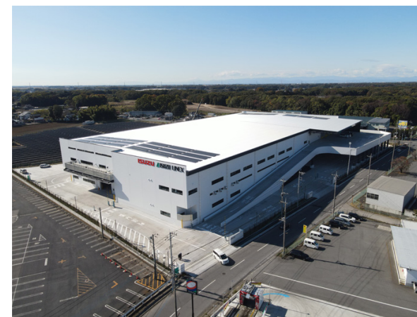
Isuzu Logistics Global Center commenced operations in April 2020
