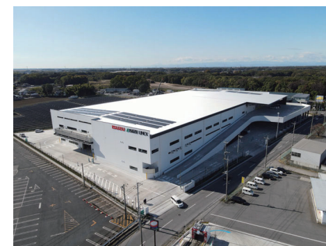
Isuzu Logistics Global Center commenced operations in April 2020
