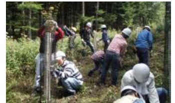
Trying hard to install netting fences with unaccustomed hands
