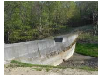
Sand control dam installed in the site
