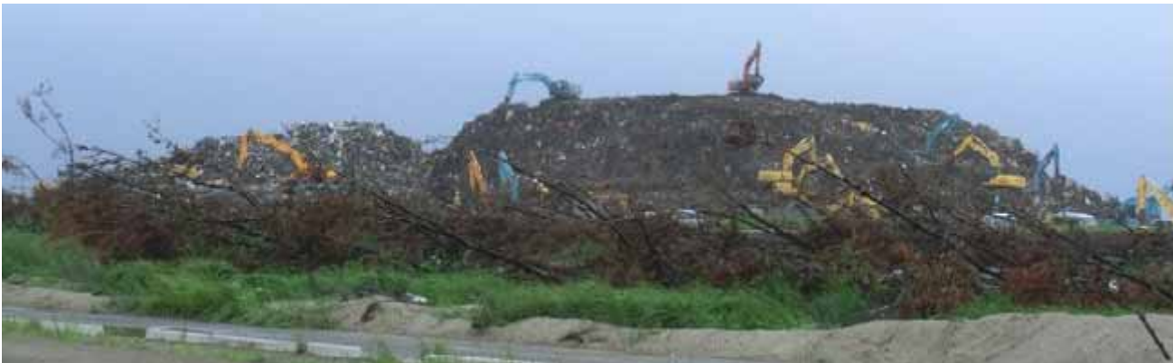
Diggers for debris removal
