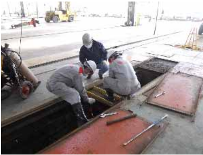
Removing the lift.
