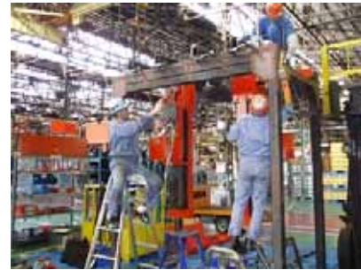
Repairing the lift.
