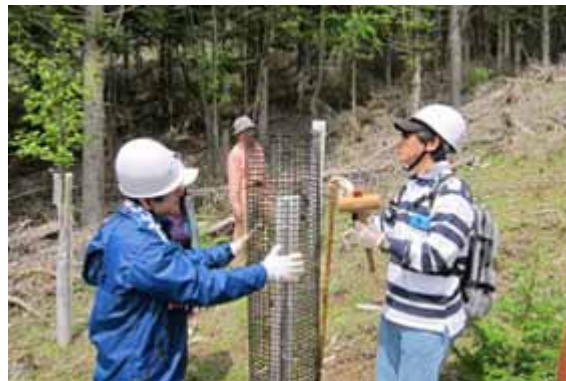
Installing netting fences to avoid harm caused by deer
