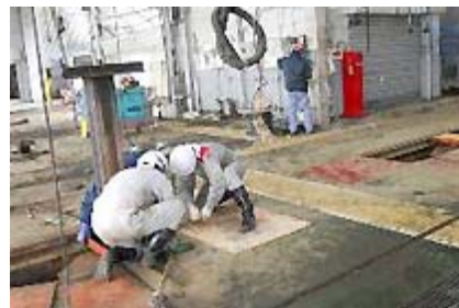
Restoration activities at service locations in disaster areas
