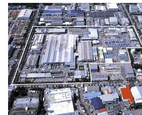
A complete view of the plant
