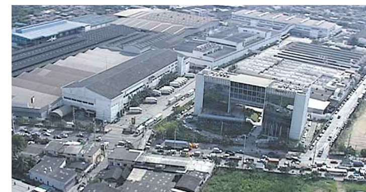
A complete view of the plant
