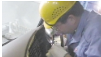
Testing the ease of dismantling interior panels
