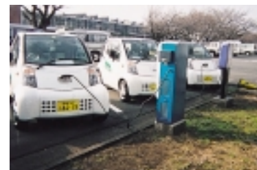
Electric vehicle parking and charging equipment
