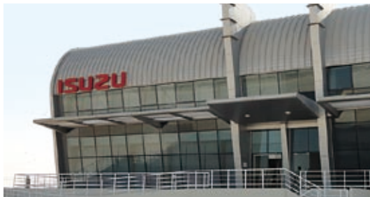
Middle East After-Sales Center office
