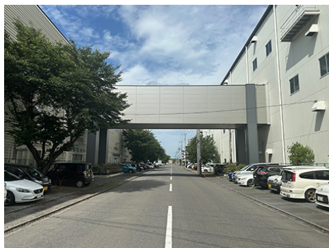
Overpass installed between warehouses
