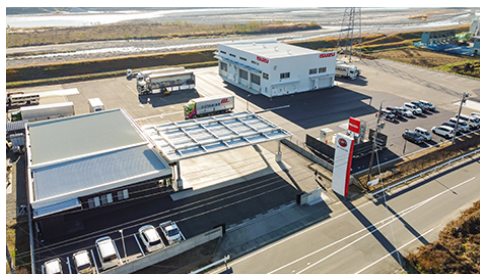
Isuzu Motors Chubu Co., Ltd. Iida Service Center
