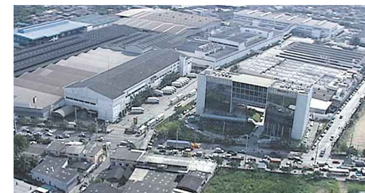
A complete view of the plant
