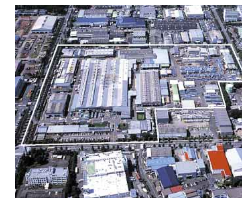
A complete view of the plant
