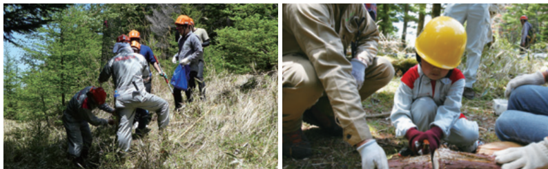
Repairing protective nets
